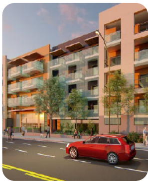
149 units in Warner Center (existing office building)
