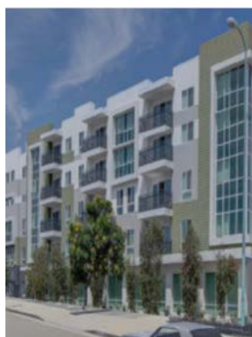
148 units in Warner Center (existing office building)
